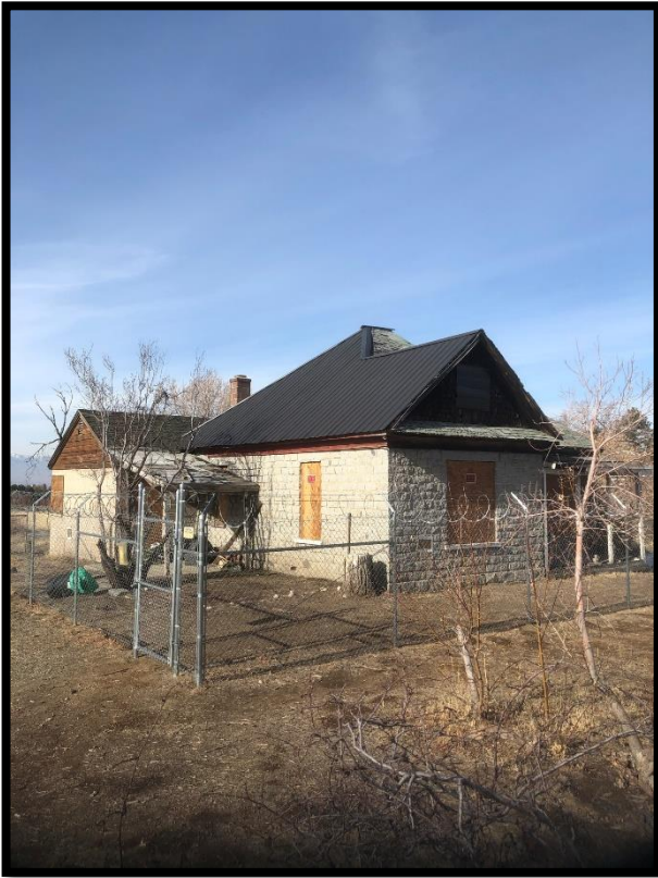
Added temporary roofing and safety fencing
