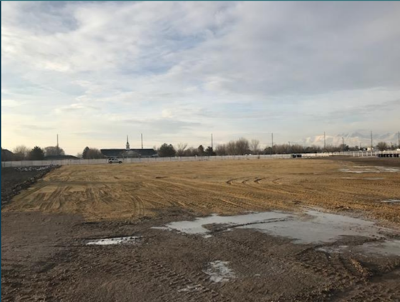
Existing retention basin removed and converted into parking area
