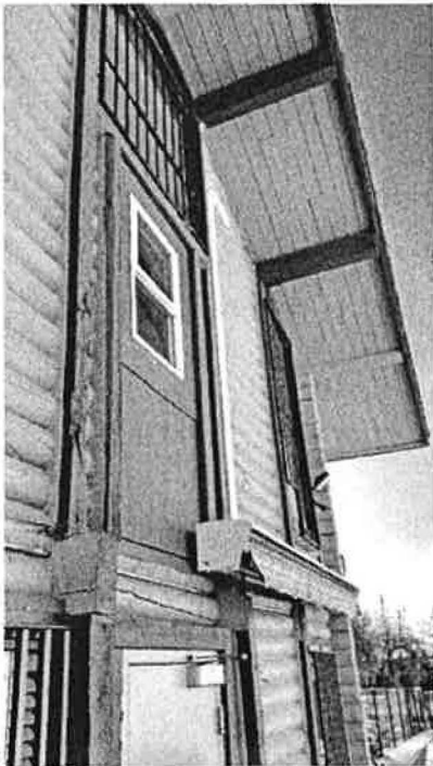
Former door leading to former balcony. Balcony had to be removed because it was no longer safe. It was termite infested. City came and removed it and blocked door.
