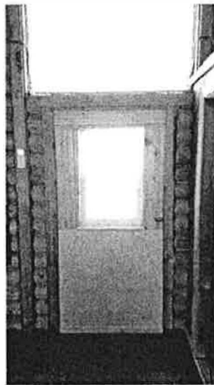
Former door leading to former balcony. Balcony had to be removed because it was no longer safe. It was termite infested. City came and removed it and blocked door.
