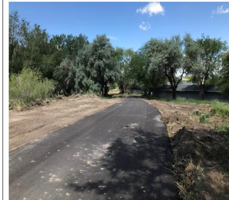
After – looking west along nearly finished trail
