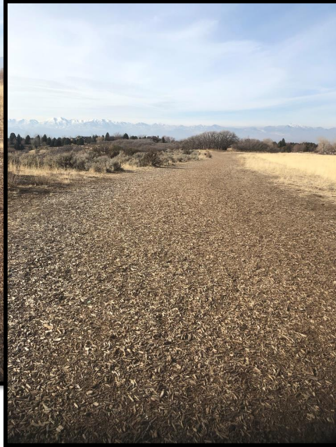
4+ miles of trail surfaced with 3,500 cubic Yards of Bark Mulch
