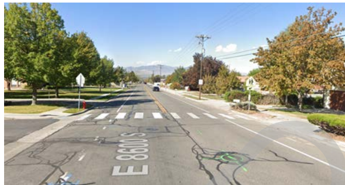
Credit: Google Maps Street View, 2021.
