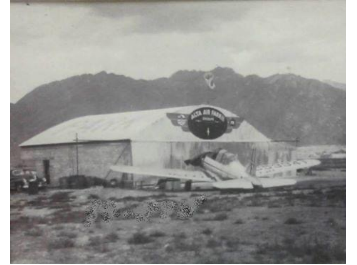
Figure 2.32: Alta Air Park.
