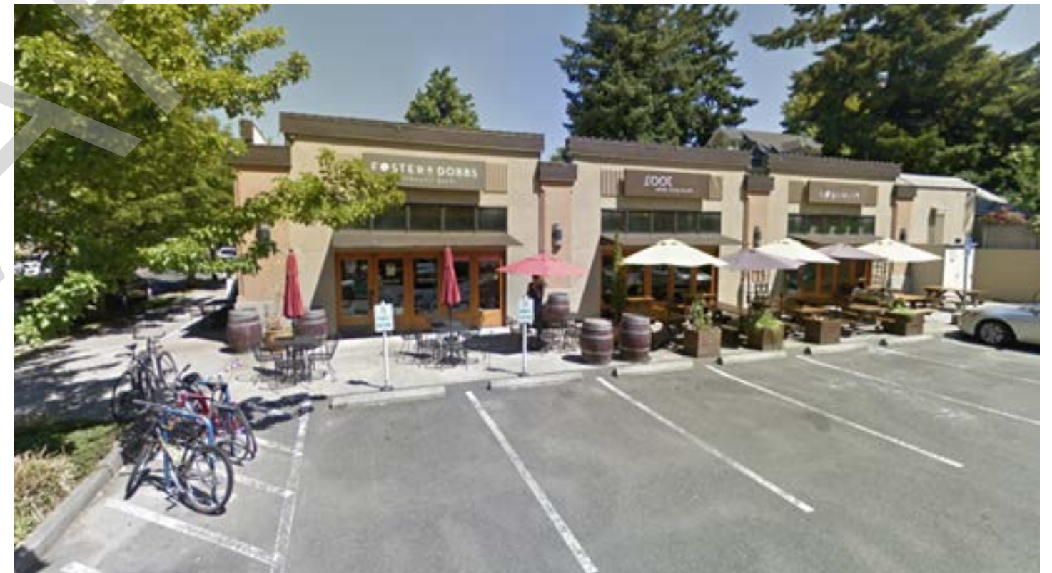
Credit: Google Maps Street View, 2017.
