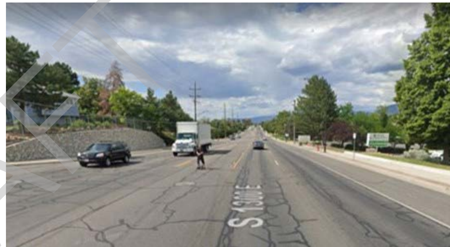
Figure 3.21: Man Waits to Cross Street on Segment of 1300 E Where Medians are Absent.
