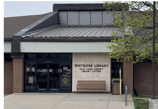
Whitmore (Cottonwood Heights) Rebuild
