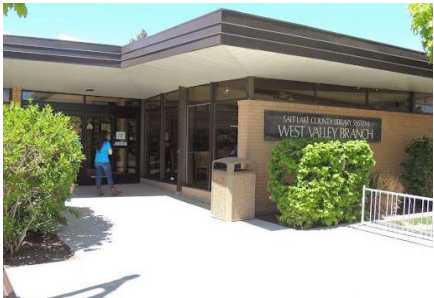
West Valley Rebuild
