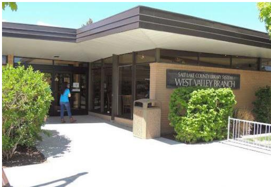
West Valley Rebuild
